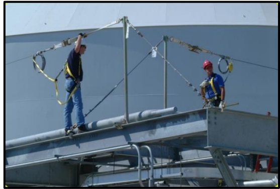
Figure 6: Horizontal life-line system
